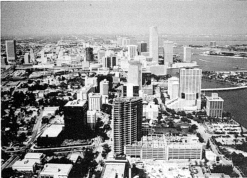
Miami's downtown business district. At left is Brickell Avenue, the city's Wall Street. Miami is now enjoying a major downtown building boom, with $1 billion in new office space under construction.
