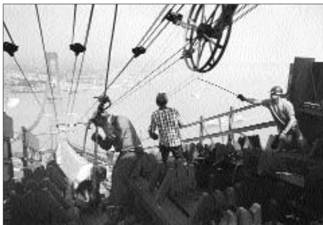
Workmen attach a cable over the tower saddle on the Verrazano-Narrows Bridge in July 1963.
