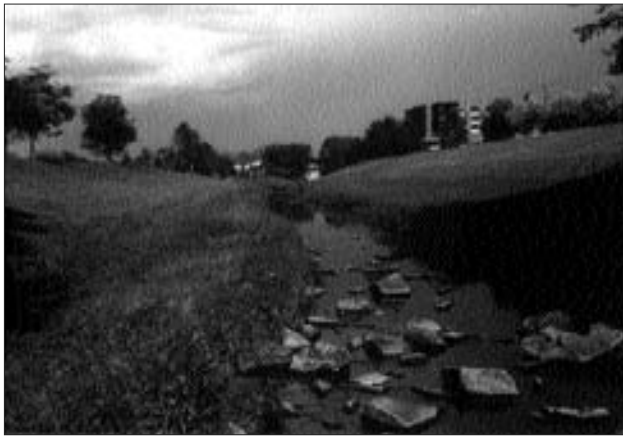
Creating a new landscape: Denver's Harvard Gulch is part of the city's Urban Stormwater and Flood Control District.
