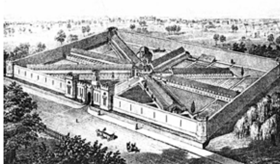
Philadelphia’s Eastern State Penitentiary combined the elements of a fortress and a monastery. All seven isolation cellblocks connected to a central surveillance hub.
