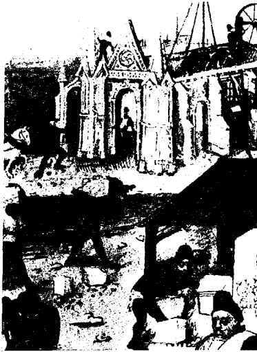
This detail from a 15th-century painting depicts the rebuilding of the west front of St. Denis Church, near Paris.
