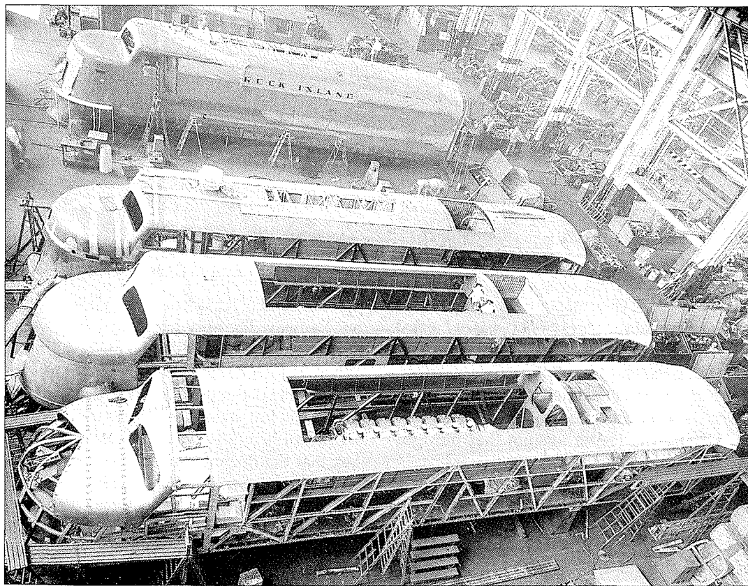
Diesel engines are installed in Rock Island Rocket locomotives at General Motors's Electro-Motive plant in La Grange, Illinois, circa 1938. The famous "E" locomotives were capable of an impressive 117 MPH.
