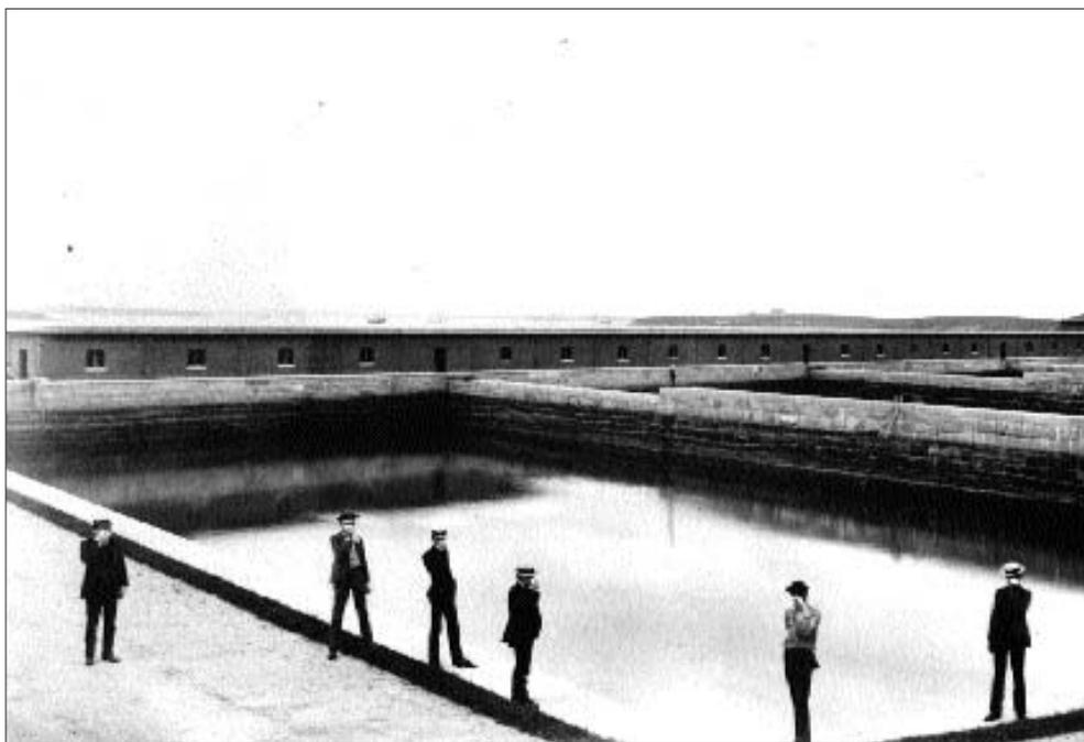
*The sewer basin on Moon Island in Boston Harbor during the 1880s, a time when a general concern with foul water gave way to a focus on the control of sewage.*
