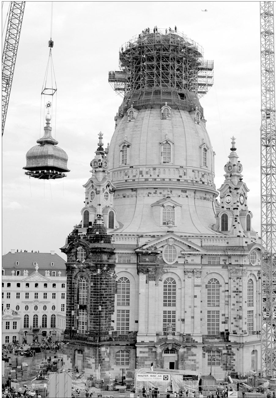
A cupola adorned with a gilded orb and cross is hoisted atop Dresden's Frauenkirche in 2004 as part of a restoration financed by charities from several countries, including Great Britain and the United States. The crowning ornaments were crafted by a team of British silversmiths, among them one whose father participated in the World War II raid that destroyed the church.
